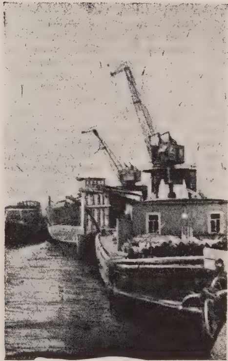
Unloading at landing stage of the Moscow-Volga canal
