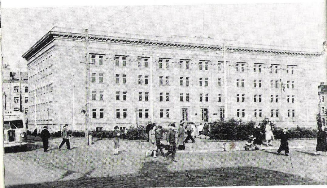
A new building for the Teachers' Training Institute in Daugavpils.
