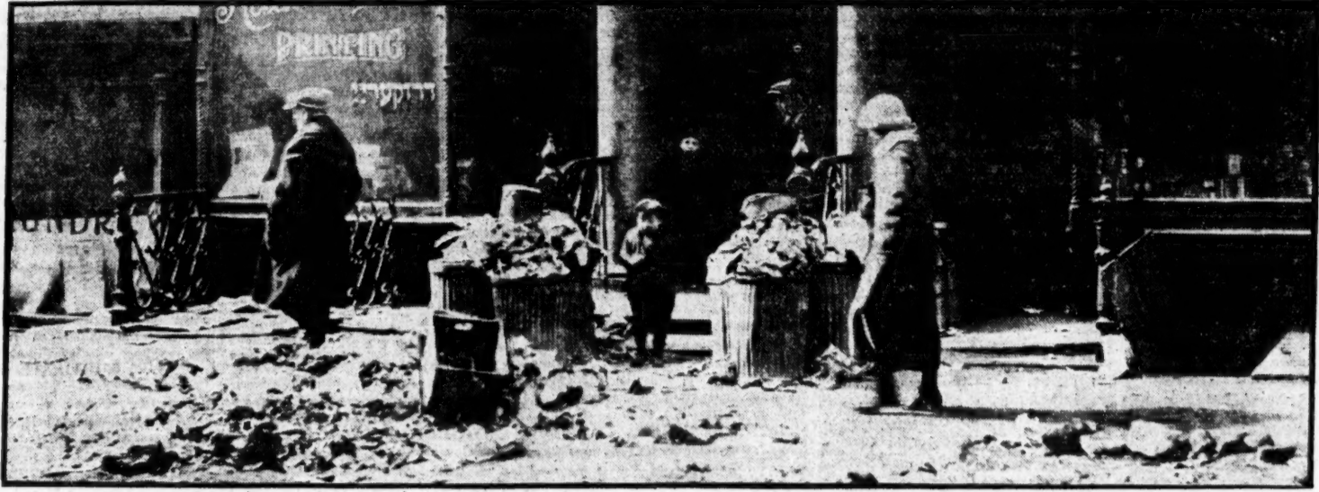
In the stifling heat of summer, when the air is poisoned by the filth of tenements, wooden rookeries and decrepit yard-houses, the New York slum dwellers pray for winter. When winter comes, the freezing inhabitants of the heatless hovels look forward to summer. Here is a winter scene of the East Side. Garbage and dung heaps mix with the snow, cluttering the sidewalks as well as the gutters. This menace to life sometimes is on the ground for weeks before it is cleaned up. Often it stays until the thaw carries it away.
