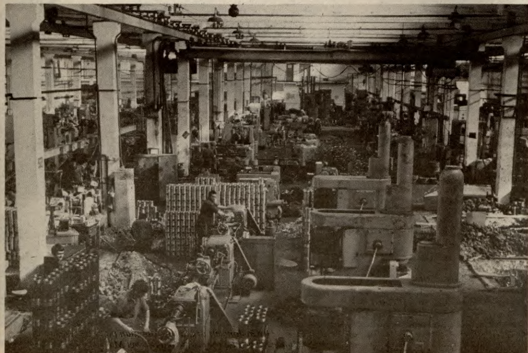
Inside the Tirana Tractor Spare Parts Factory, built on the basis of extensive Chinese aid.
